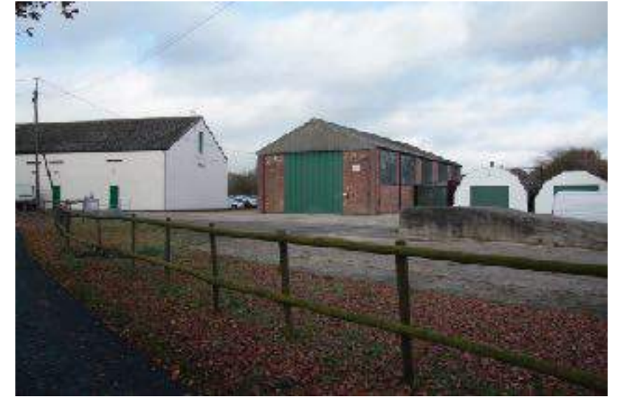
P3 - Coldstore, shelters and industrial units to be demolished
